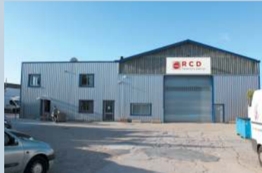
PMG RCD - New building
